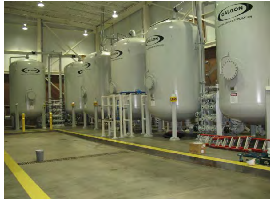
Carbon treatment systems to treat PFAS in water (MDH, 2012)
